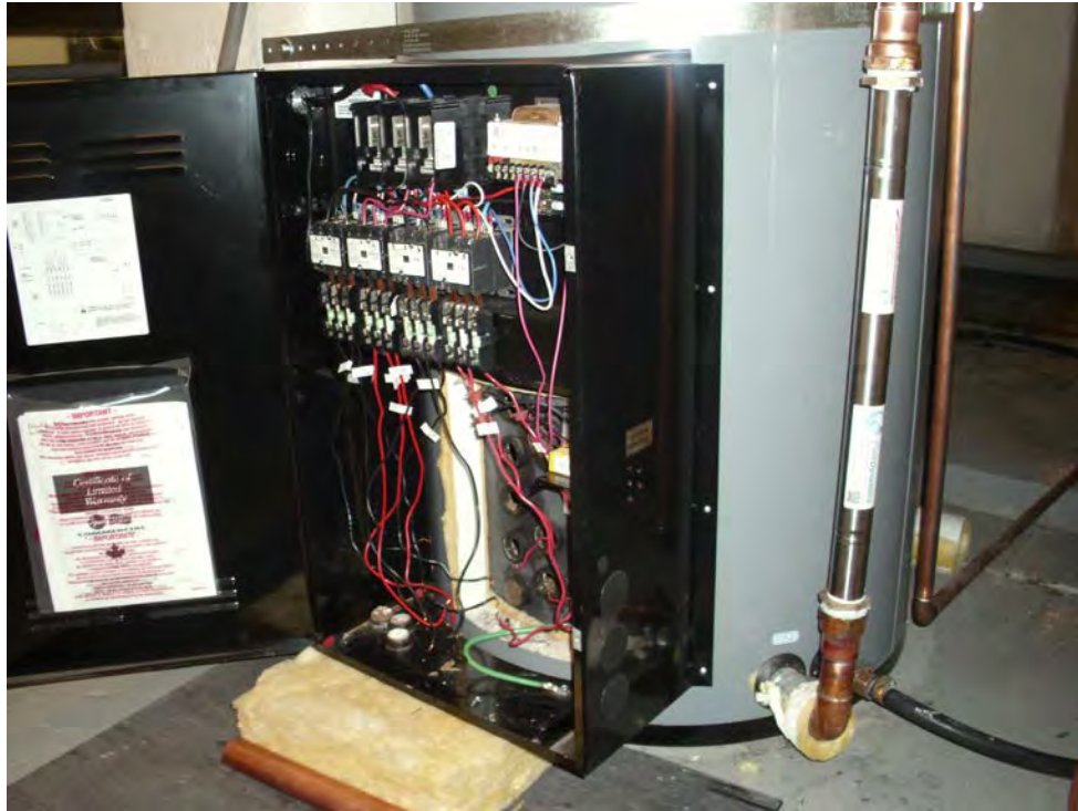
Figure 6. Final Configuration for the Nonchemical Water Treatment System (silver section of pipe on the cold water inlet to the water heater tank).
